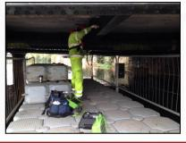
The inspection was carried out over two days and included a detailed inspection of the piers and soffit steelwork and the parapets. Adhesion testing, dry film thickness measurements and the analysis of the existing coatings was carried out. A detailed report based on the findings from the survey was then provided to the client with recommendations for maintenance work and repair procedure in line with Highways Series 5000 Maintenance Painting of Steelwork.
