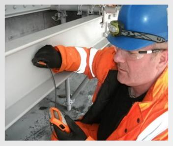
The SOBI Benchmark Testing requires a detailed survey of the structure as follows: Carry out an assessment in line with BD87/05 along with collecting paint samples for review of hazardous content and assessment of coating type and adhesion testing to identify the tensile strength of the coating system.
